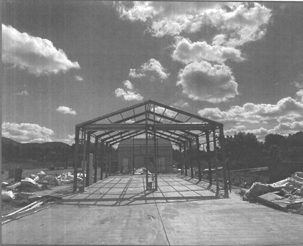
Station 2 engine bay removal progress
